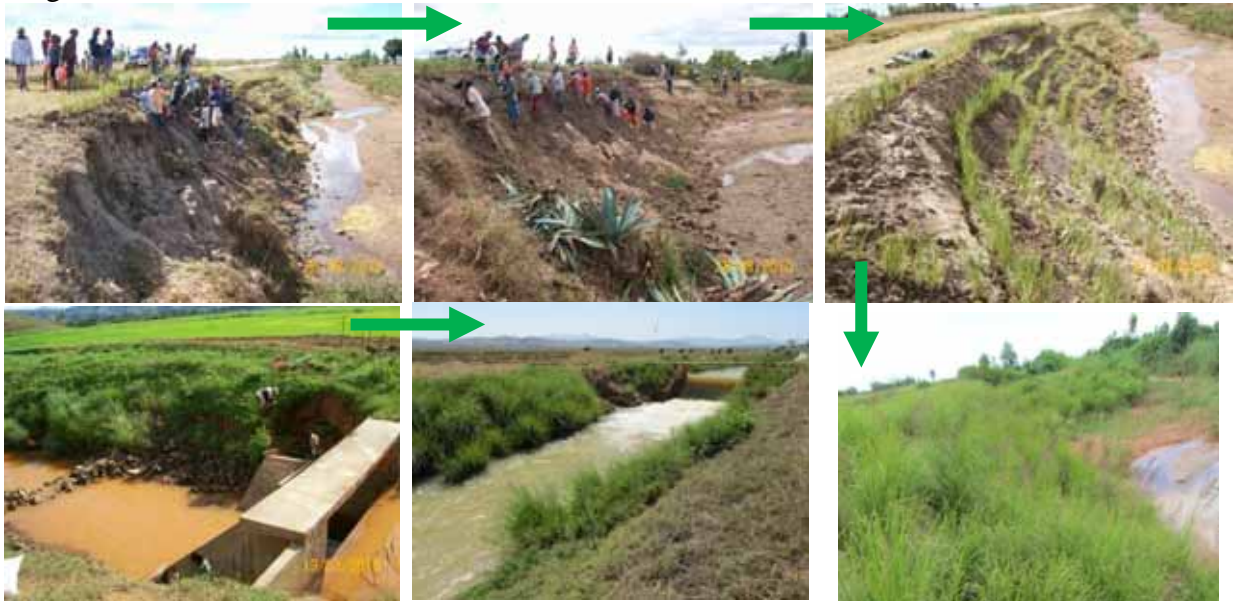
Transplantation of VHR for Banks Protection
